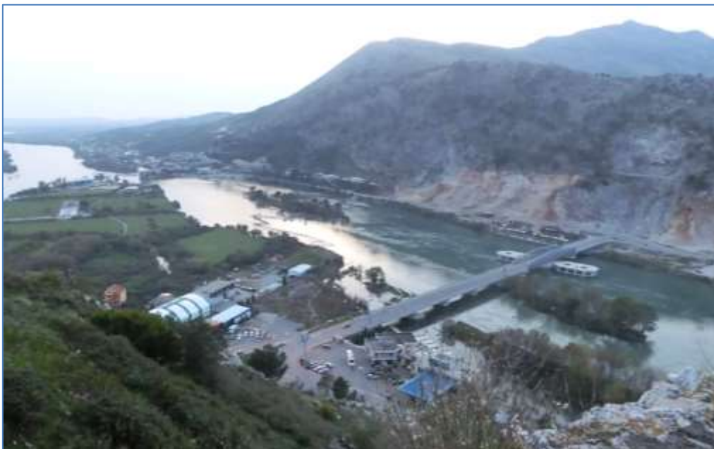
Figure 20: View on the New Bridge connecting SH1 and SH41 to the Montenegrin Border [photo: INFRASTRUKTUR & UMWELT]
