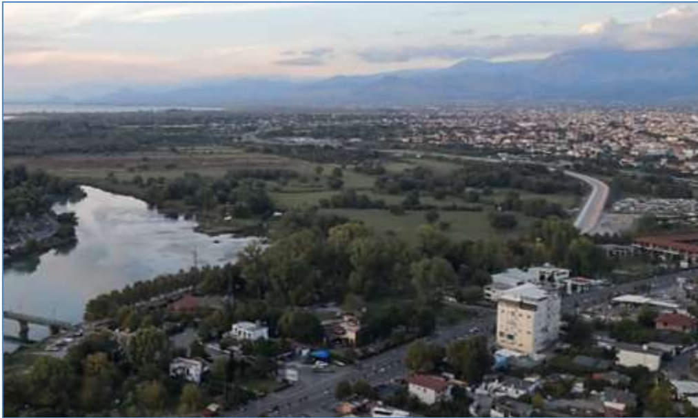
Figure 19: View on the Western Bypass (under construction) of Shkodër City [photo: INFRASTRUKTUR & UMWELT]
